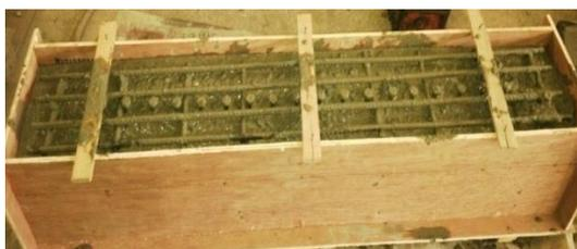
Fig. 2 Formwork, reinforcement, studs welded to steel beam and a layer of concrete being vibrated during casting
